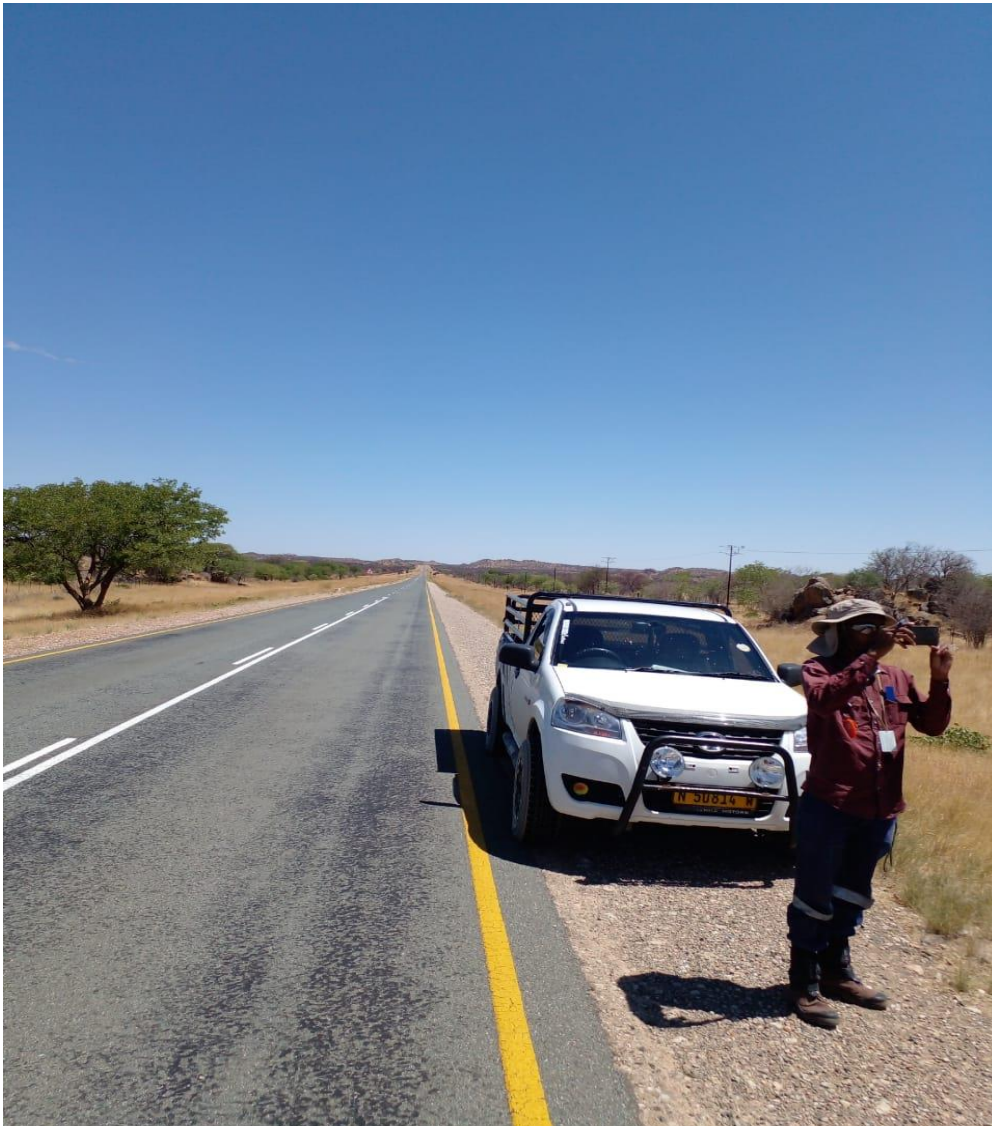
Figure 5-Access & Tarred road that cuts through EPL 7125.
